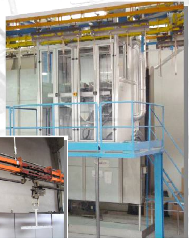
Paint removal in a Power&Free conveyor system
